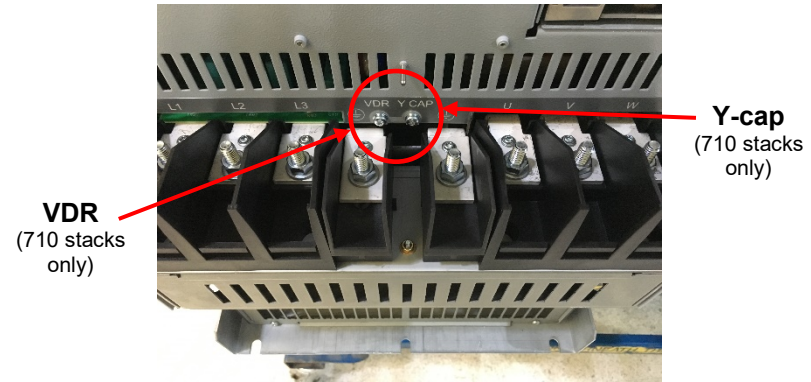
Bottom Terminal Area
